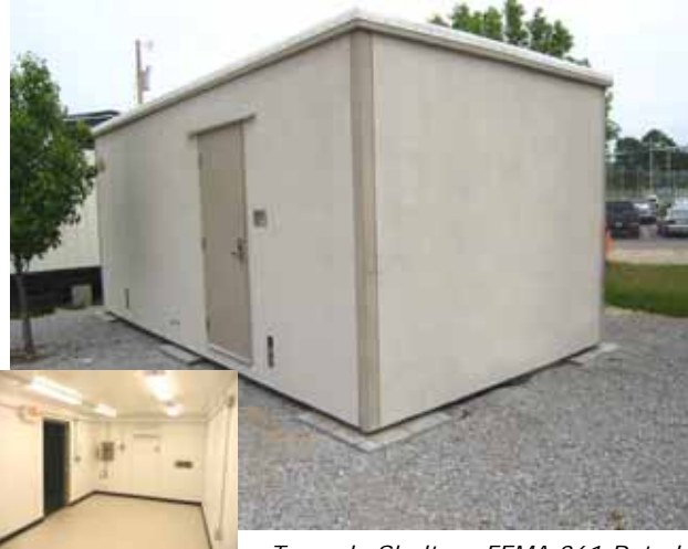
Tornado Shelter—FEMA 361 Rated
