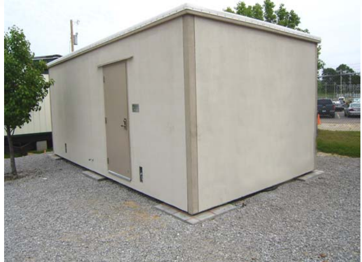
30 Person Occupancy FEMA 361 Rated Community Safe Room
