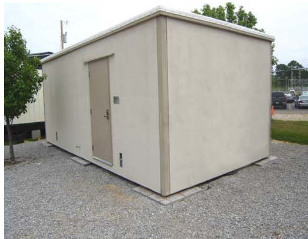
Custom FEMA 361 Rated Community Safe Room
