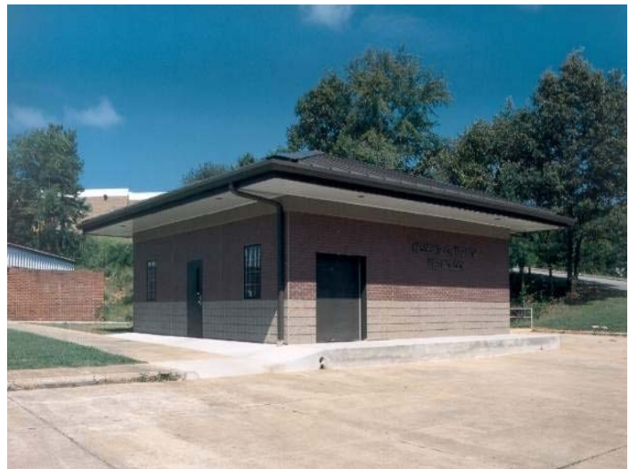
Concessions & Restroom with Stick Built Roof
